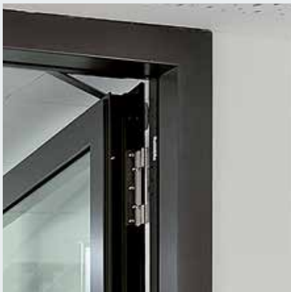
Frame prepared for overhead door closer
